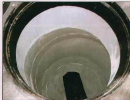
In corrosive environments, a manhole can be replaced without digging by installing a plastic liner fitted to a form, and filling the annulus space between the form and the old wall with concrete.
